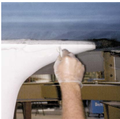
Fig. 13 The joint is tooled off and finished
