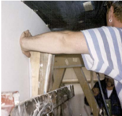
Fig. 11 A keel is carefully slid into position
