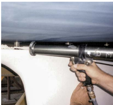
Fig. 12 The adhesive is applied
