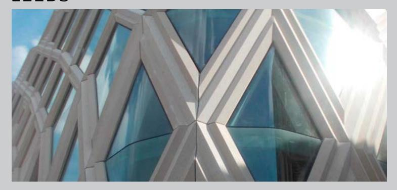
Sikasil® SG-500 has been used to bond 192 windows – a mix of 1m x 2m and 5m x 3m windows – to diamond-shaped steel frames which form the 25,000m² building's five-storey, three-dimensional façade, described by specialist retail developers Hammerson as a "future classic for architecture in Leeds".
