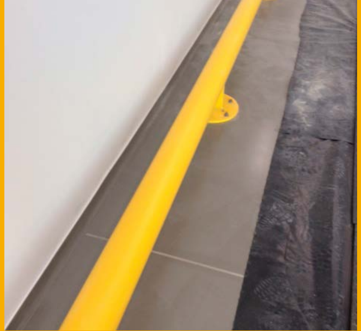
Finished floor and cove junction
