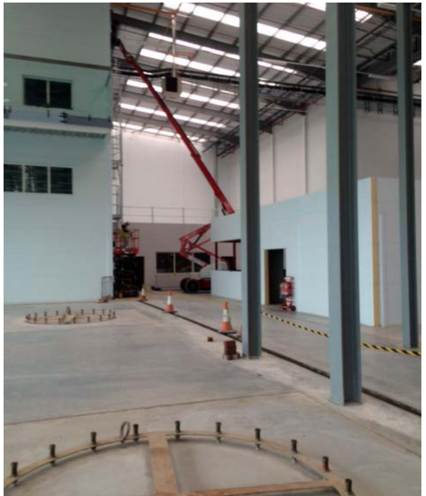
↑ Issues with drains on arrival on site being set level with existing concrete substrate and channel running out of tolerance either side of the linear meter frame.
