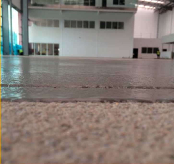
Upside down Sika Purcem HS21 scratch coat primer
