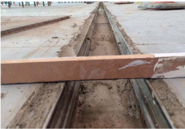
← Diamond grinding surface preparation of C40 concrete required to remove 5 mm x 1 meter away from either-side of the drain channels in order to create edge to terminate Sika Purcem HS21 without creating an irregular visual fall back to channel
