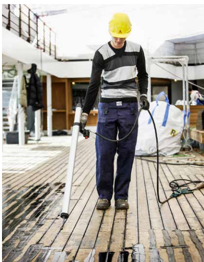
Fig. 17 Applying Sikaflex®-290 DC PRO
