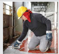
Fig. 8 Spreading the SikaTransfloor®-352 (SL/ST)
