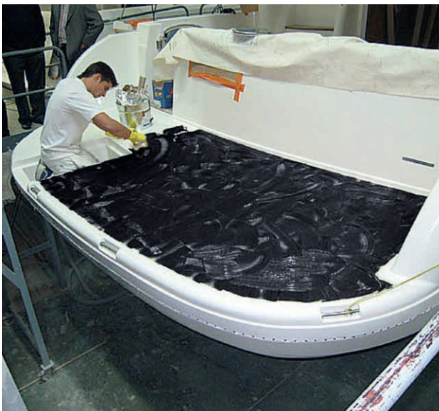
Fig. 26 Application of Sikaflex®-298
