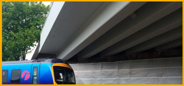
The concrete bridge, built in 1964, displayed major signs of carbonationinduced spalling to columns and deck soffits above the rail lines. Contractors, BOSA Contracts, on behalf of Hull City Council, required a practical repair solution which extended the lifespan of one of the city's arterial routes without impacting on daily road and rail commuter journeys or impeding pedestrians.
