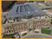
SINGLE PLY ROOFING
