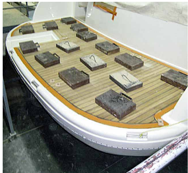
Fig. 27 Holding in place with weights
