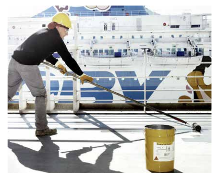
Fig. 3 Applying SikaCor® ZP Primer with a roller
