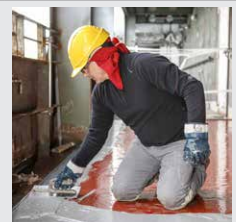
Fig. 8 Spreading the SikaTransfloor®-352 (SL/ST)
