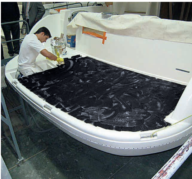
Fig. 26 Application of Sikaflex®-298
