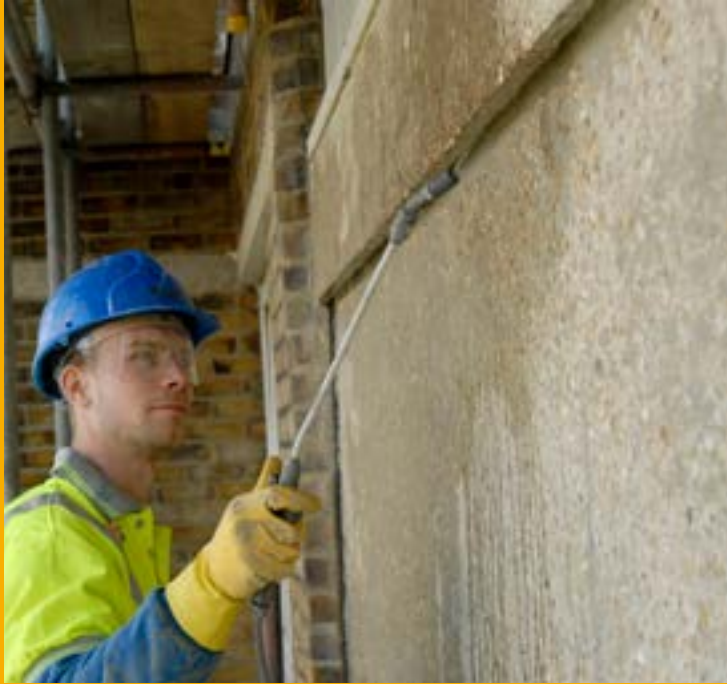
Example of Sika® Ferrogard® being installed
