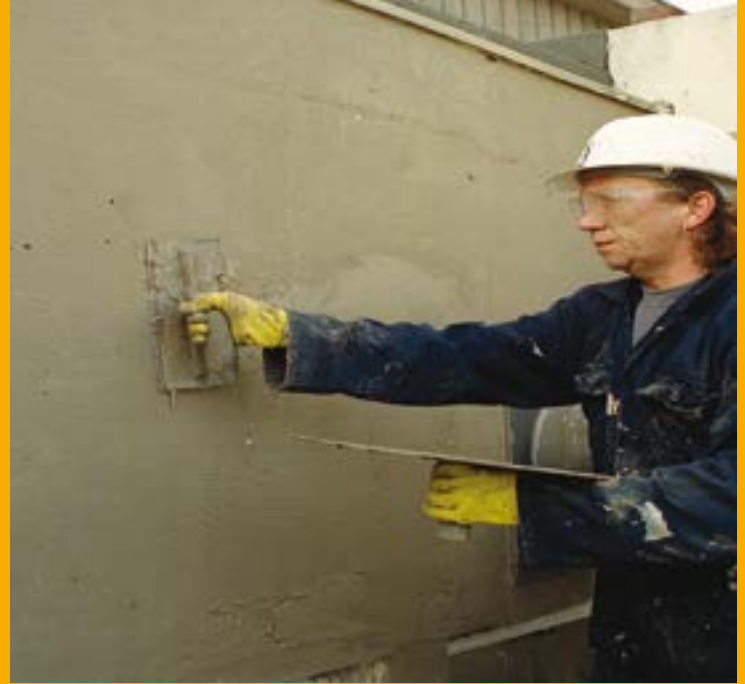
Example of Sika® MonoTop® being installed
