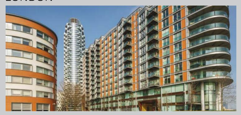
Contractors, Lindner Façades, specified SikaMembran® for two blocks - a 44-storey private residential tower and a 12-storey affordable housing, mixed-use development – using the system to create an air and weathertight seal around an estimated 22,000m² of façade.
