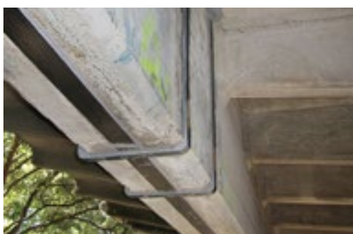
Sika CarboDur® strips and CarboShear L plates bonded to the concrete structure.
