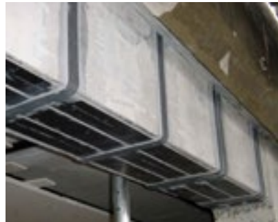
BEAM STRENGTHENING
