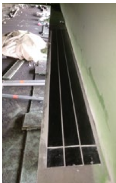
Two layers of Sika CarboDur®
