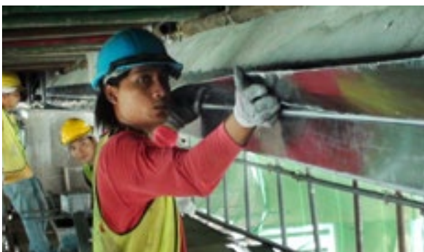
Installation CarboDur®
