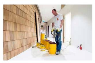
**STEP 1.** After inspection and preparation of the subfloor by cleaning (and if needed shotblasting, grinding, sanding and/or leveling), we will start mixing our liquid materials.
