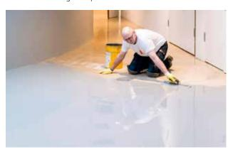
**STEP 3.** Self-leveling materials are applied in one or several layers to create a seamless base. Experts will pour and distribute the liquid material by using special squeegees, hand trowels, stand-up trowels and spike rollers in the process to assure a perfectly even and smooth surface.
