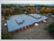
LIQUID APPLIED ROOFING
