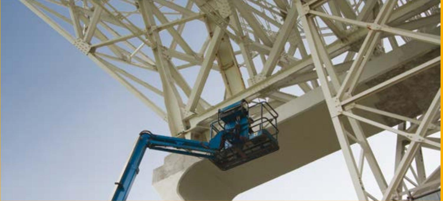
Supporting the 25x38 metre diameter telescope dish, the concrete frame stands 25 metres high and was constructed fifty years ago. To make primary repairs, Grade 2 utilised cherry pickers to apply the two-component Sika® MonoTop® system – comprising a bonding primer and reinforcement coating followed by a concrete repair and reprofiling mortar.
