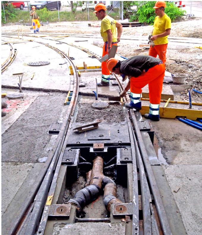
Urban planners are obliged to expand local public transport to cope with the rapid development of urban spaces. This trend requires a reduction in vibrations and noise in the rail fastening system, therefore the flexible and volume-compressible grouting materials become the effective, long lasting solution.
