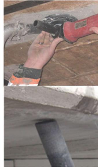
The mechanical preparation is carried out to remove cement laitance, any loose and friable materials and achieve a profiled, open textured surface. Any surface defects such as honeycombing, blowholes and voids must be fully exposed.
