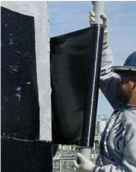
Either impregnate the whole pre-cut fabric strip or cut the fabric after the desired length is saturated.
