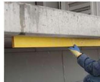
The final surface must be smooth, dry and free of damaged concrete and any other contaminants as dust, foreign particles, cement laitance, oil, grease, surface coatings, curing compounds, waxes and impregnations etc., which could adversely affect or inhibit the bond of the strengthening system to the concrete.
