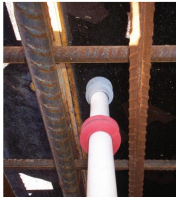
There are different materials, products and methods used to seal the waterproofing details. Besides the swellable products, the post-applied bonded tape Sikadur®-Combiflex® SG System is a reliable and easy-to-apply sealing solution for such details and creates a closed waterproofing system.
