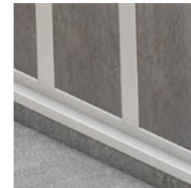
Connection joints between precast concrete elements need to be sealed after installation of the individual segments. In addition, all transitions/connections to in situ concrete must be sealed – typically using the Sikadur®-Combiflex® SG System.
