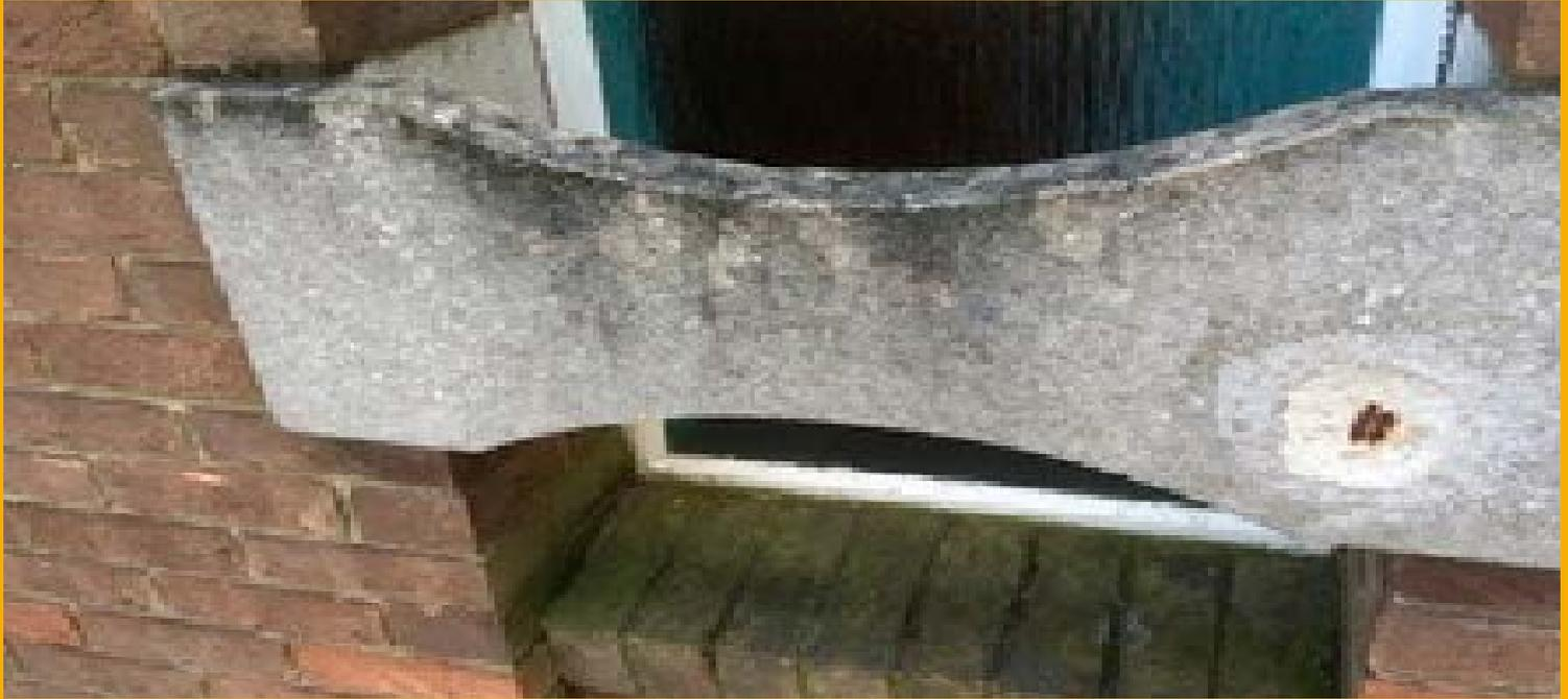
To make good the damage and eliminate the risk of future corrosion in the spalled areas, [Sika® MonoTop®](#), a proven, high-performance concrete repair and protection system, was specified.
