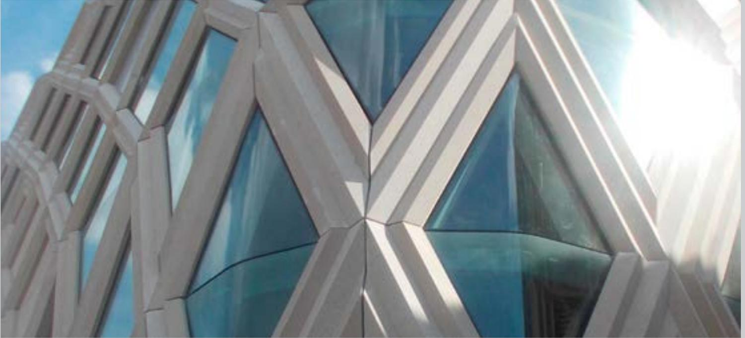
[Sikasil® SG-500](#) has been used to bond 192 windows – a mix of 1m x 2m and 5m x 3m windows – to diamond-shaped steel frames which form the 25,000m<sup>2</sup> building's five-storey, three-dimensional façade, described by specialist retail developers Hammerson as a “future classic for architecture in Leeds”.
