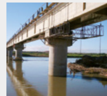
Ernest Oppenheimer Bridge (ZA)
