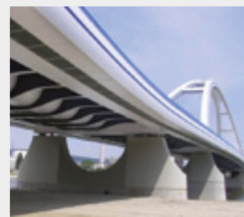
Apollo Bridge, Bratislava, (SL)
