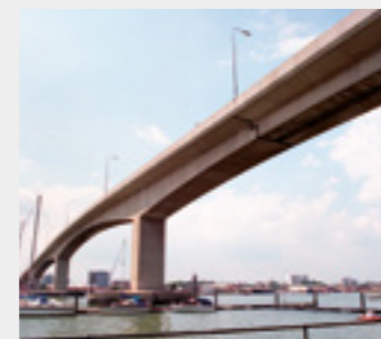
Itchen Bridge, Southampton (UK)
