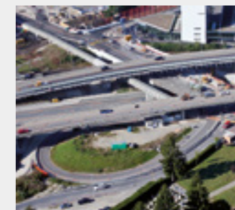
Highway Bridge A1, Bern (CH)
