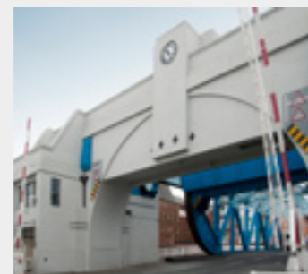
North Hull Bridge (UK)
