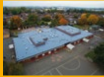
LIQUID APPLIED ROOFING
