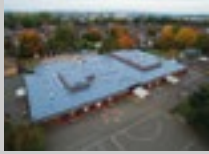
LIQUID APPLIED ROOFING
