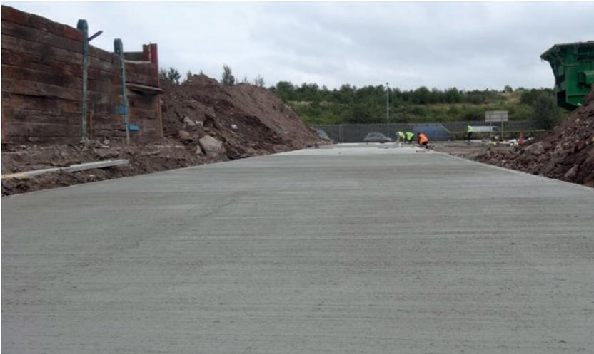
Oakfield recycling centre in Hucknall needed a concrete slab that could withstand the impact of heavy machinery to replace their existing steel mesh system. The use of SikaFiber® Force synthetic macro-fibers delivered the strength required while also eliminating the risk of corrosion and other issues associated with traditional steel reinforcement.
