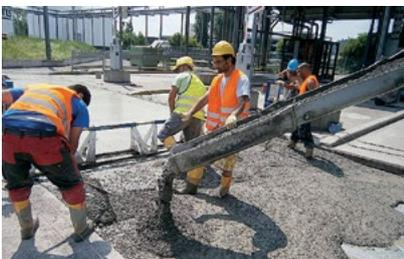
SikaFiber® Force synthetic macro-fibres were used together with the German 'white-topping' method for repairing the slabs in an oil harbour in Stuttgart. The fibres were used to improve the fatigue behaviour of the new concrete topping.
