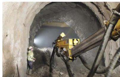
SikaFiber® Force synthetic macro-fibres were added to the sprayed concrete to increase the ductility of the concrete lining. This kind of fibre-reinforced concrete produces a more efficient and cost-effective excavation support.
