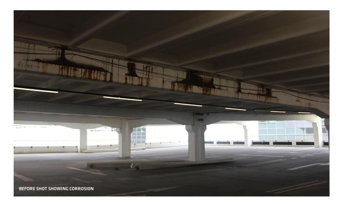
The Purple and Green MSCPs have capacity for more than 4,000 vehicles across five levels. The project's scope involved concrete repair, structural strengthening using carbon fibre laminates, the replacement of the conduits, movement joints, drainage channels and deck waterproofing.
