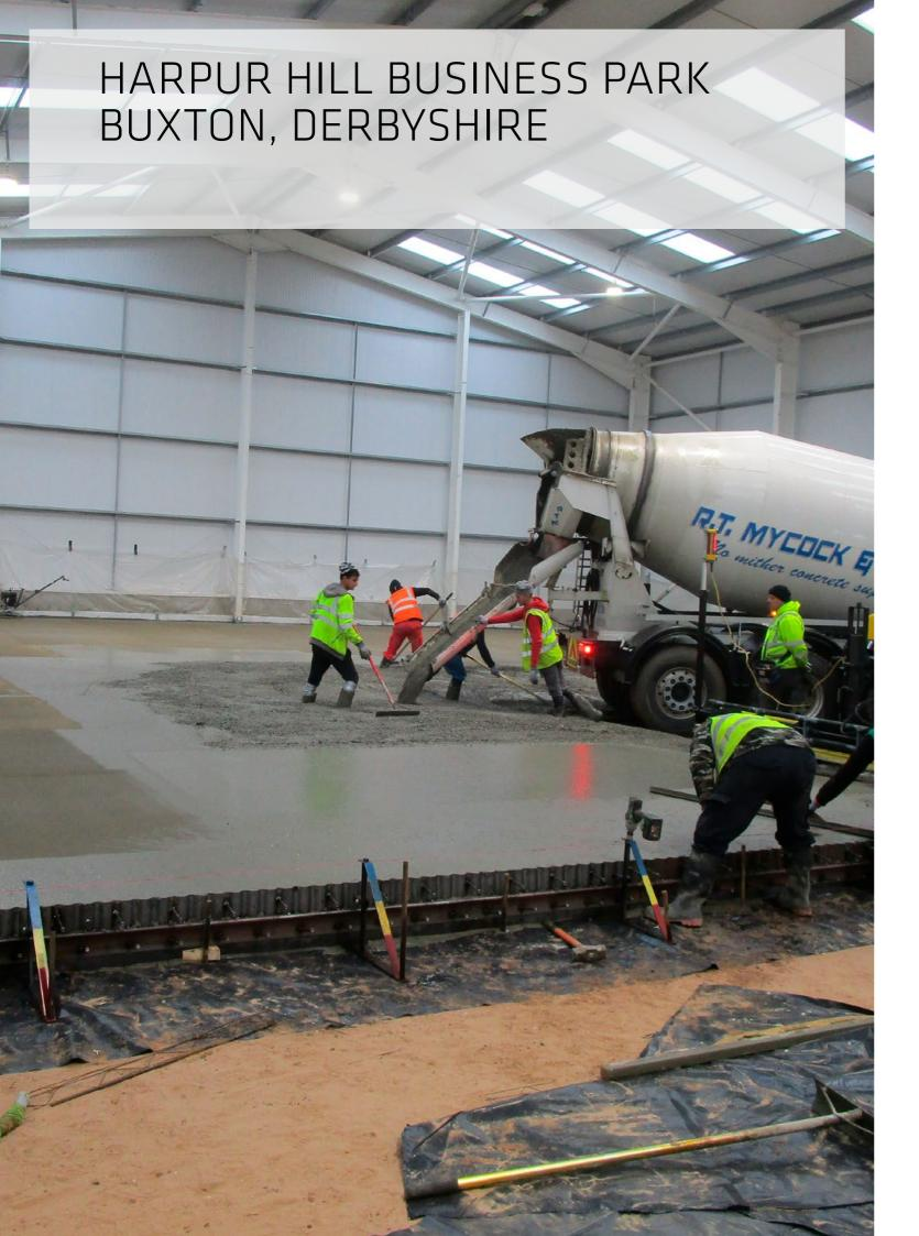
SIKA'S STRENGTH USED IN CONCRETE SLAB FOR WAREHOUSE BUILDING. Specification and installation of a concrete slab within a 4,000m² warehouse on the Harpur Hill Business Park in Buxton, Derbyshire.
