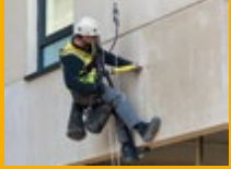
JOINT SEALING
