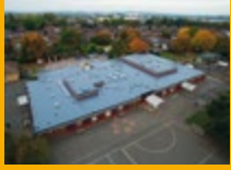
LIQUID APPLIED ROOFING
