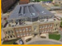
SINGLE PLY ROOFING
