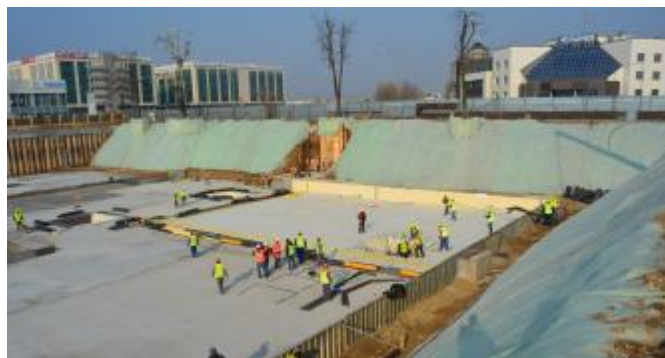
Open-cut, sloped excavation
