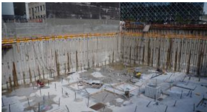
Vertical excavation, e.g. piled walls
