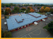
LIQUID APPLIED ROOFING
