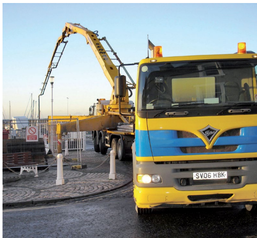
Pumping concrete from the harbour side
