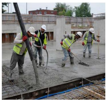
Sika® Watertight Concrete has a long and successful track record and meets BS 8102 grade 3 protection for ventilated residential and working areas.
