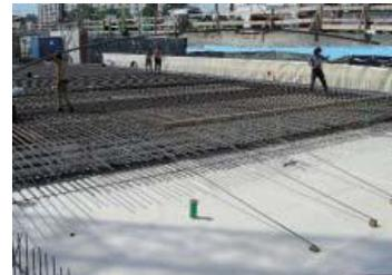
Due to the requirement of full-surface bond, the steel reinforcement must be fixed carefully on the membrane using appropriate spacers.
