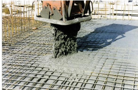
The concrete quality is a key factor for a durable and successful waterproofing system. It enables a full-surface and permanently bonded solution, without any lateral water migration between the **SikaProof® A+** membrane and the concrete structure.
