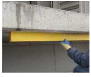
The final surface must be smooth, dry and free of damaged concrete and any other contaminants as dust, foreign particles, cement laitance, oil, grease,
