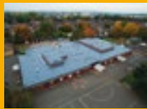
LIQUID APPLIED ROOFING
