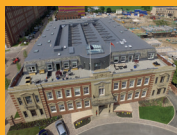
SINGLE PLY ROOFING
