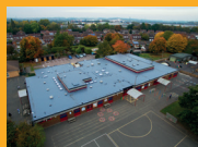
LIQUID APPLIED ROOFING
