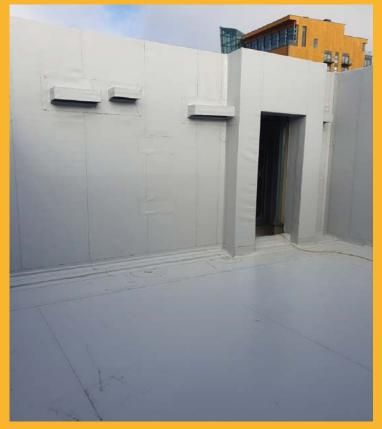
Before the roofing contractor approached the zig-zag upstand, the main flat roof was installed, cutting around it and installing peel stops. Flashing was cut to fit the area and, once the vapour barrier was fastened to the timber substrate, S327-15EL single ply in light grey was installed with fixings and finished with a drip-edge trim.
