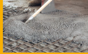
CONCRETE AND REPAIR
