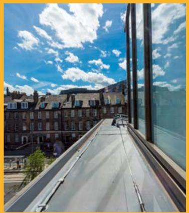
The 2mm thick Trocal S membrane was mechanically fixed using Sika-Trocal's innovative laminated metal disc system. This system sees the membrane and insulation mechanically fixed to the roof in a single process, ensuring a fast installation minimising components required and reducing overall project costs.
