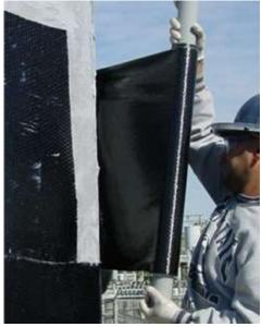
Either impregnate the whole pre-cut fabric strip or cut the fabric after the desired length is saturated.
