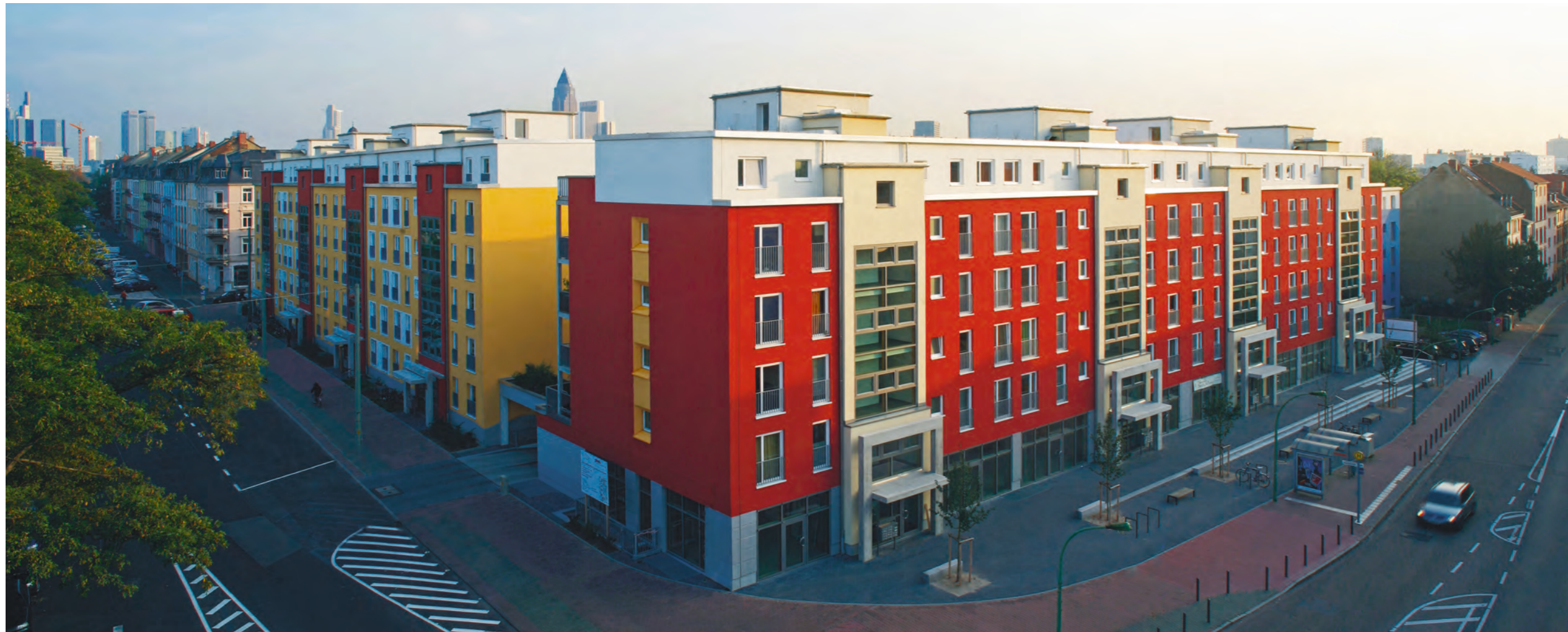
Bottom: Modern passive house in big city
