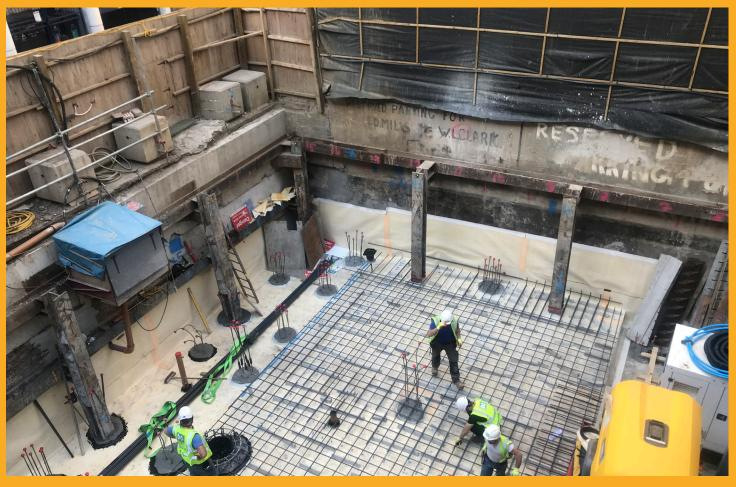
On completion, the basement was used as the site accommodation, meaning the temporary site cabins could be removed from the location to free up space. Props were left in place to allow the ground floor to be used for storage and deliveries.
