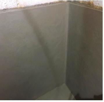
Bagged Waterproofing System, a multi-layer, mortar-based waterproofing render system with integral pore-blocking admixtures, was then successfully applied.
