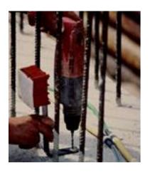
For storing the vent ends, drill a hole into the bottom of the junction box.
