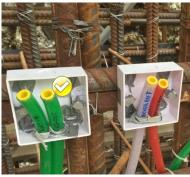
Check if total system length of the SikaFuko® injection hose is correct and as defined in Section 9.4.
