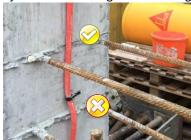
• The injection hoses should not be visible after concreting; only the PVC vent ends are to be visible.
