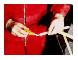
Slide the *SikaFuko*® injection hose over the *SikaFuko*® connecting nozzle and fit together so as to create a tight connection.
