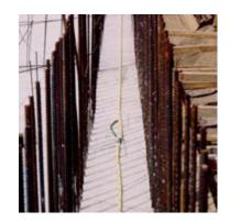
Drill holes for the *SikaFuko®* hose clips installation. Drill bit of diameter 6mm for the clips supplied in the Combi-Pack box are necessary.
