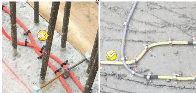
Check the placing and positioning of the SikaFuko<sup>®</sup> injection hose system The injection hose part needs joint contact along its entire length.
