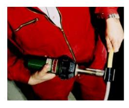
The  $SikaFuko^{\circ}$  injection hose is ready for installation after closing the vent ends with the  $SikaFuko^{\circ}$  closure plugs.
