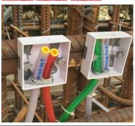
To avoid any movement or slippage, tie the vent ends with cable binders at the metal bracket. The installation of the assembled *SikaFuko®* system is now ready.
