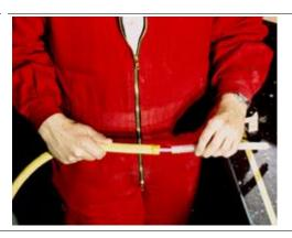
Install the *SikaFuko* heat shrink-seal sleeve in the middle, covering the connection between the PVC-vent end and the *SikaFuko* injection hose...
