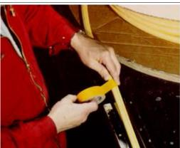
Cut the SikaFuko® VT 1 SikaFuko® VT-2 or SikaFuko® Eco 1 injection hose to the desired length with heavyduty cutters.
