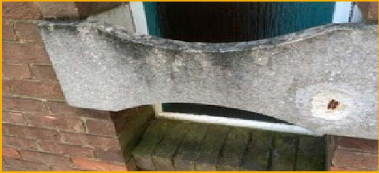
To make good the damage and eliminate the risk of future corrosion in the spalled areas, <u>Sika® MonoTop®</u>, a proven, high-performance concrete repair and protection system, was specified.
