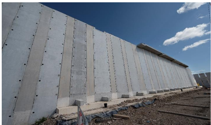
Sika® Watertight Concrete and precast concrete during construction
