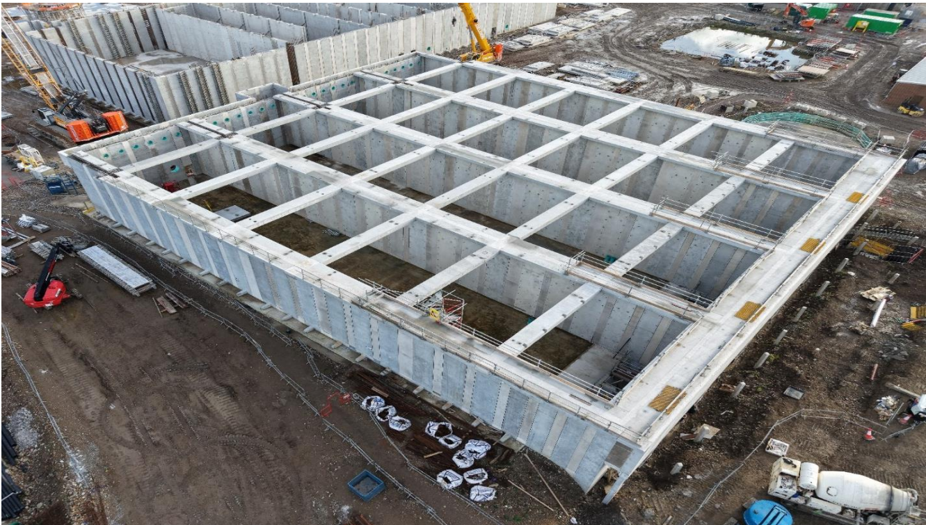
Sika® Watertight Concrete and precast concrete completed
