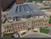
SINGLE PLY ROOFING
