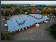
LIQUID APPLIED ROOFING
