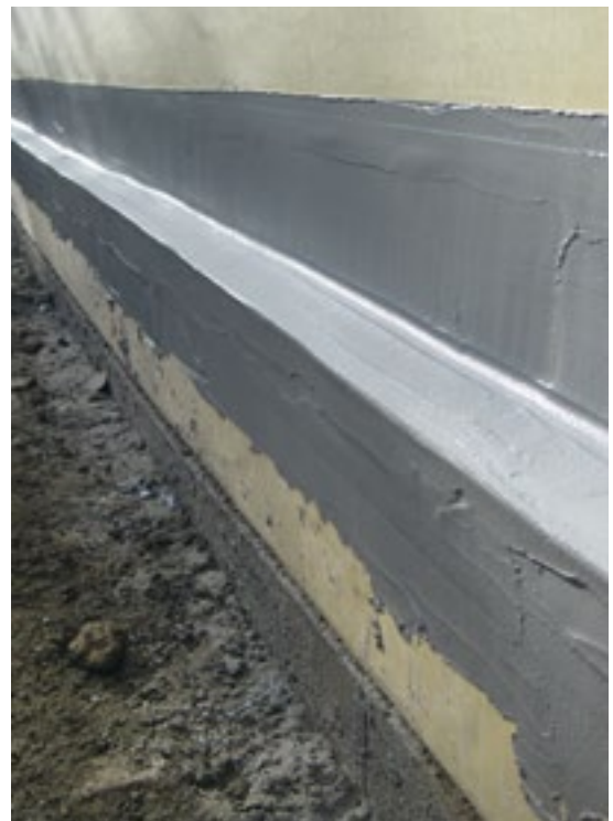
Transitions as detail solution: Sikadur-Combiflex® TF System on SikaProof® complete system
