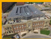
SINGLE PLY ROOFING
