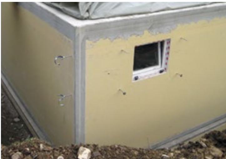
Transitions as detail solution: Sikadur-Combiflex® TF System on SikaProof® complete system
