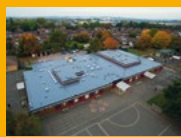
LIQUID APPLIED ROOFING
