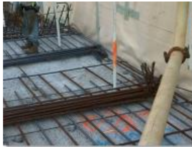
Dewatering system with temporary pipe penetrations.
