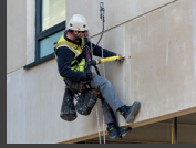
JOINT SEALING
