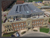
SINGLE PLY ROOFING
