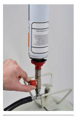
5. Aim the spray-gun into a waste container, apply pressure to the trigger on the gun to push Sika® Spray Cleaner trough the hose and gun until the adhesive starts to dispense. Keep pressure on the trigger until the hose and gun are thoroughly cleaned.
