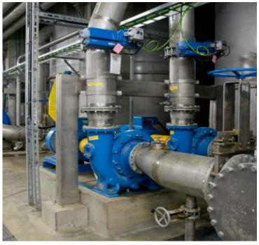
Sika® Control 40 was also used in the mix for a variety of concrete machinery bases, where the machine mounting plates were bedded into the concrete. Low shrinkage in the concrete was again required to retain the integrity of the plates.
