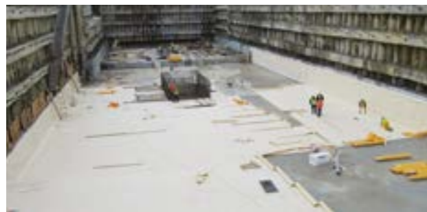
Vertical excavation wall – a typical use for SikaProof®-A under the raft and at the walls.
