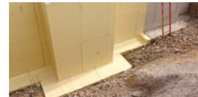
Open excavation with protrusion slab to wall, here the complete structure could be simply sealed with SikaProof®-P.
