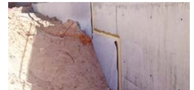
For open excavations the protection of the SikaProof® membrane is very important, especially due to the backfilling.
