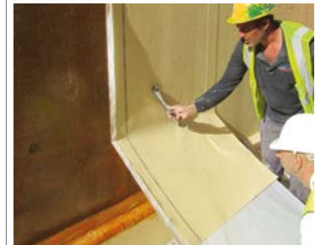
THE SYSTEM BUILD-UP SikaProof®-P has an FPO membrane (1) based on Sikaplan® technology and is supplied 0.6mm thick. It is coated with a unique Sika adhesive sealant (2), and protected with a peel-release film (3). The hardened structural concrete substrate (5) should be prepared and primed with SikaProof® Primer-01 (4).
