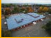
LIQUID APPLIED ROOFING
